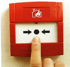
Many premises use manual call points to raise the alarm.
