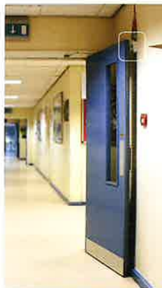
A wall-mounted magnetic fire door holder will release the door when the fire alarm activates.
