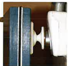
A wall-mounted magnetic fire door holder will release the door when the fire alarm activates.
