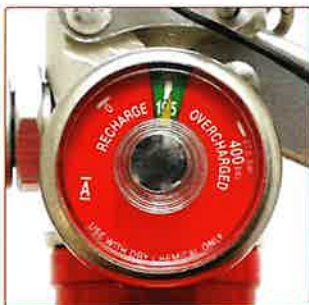
Fire extinguisher pressure gauge showing the correct pressure.
