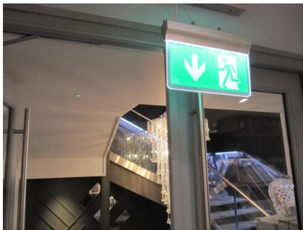
The above sign indicating a fire escape route leads to a unprotected staircase. (No protection offered if fire was on floor below) also glazed panels are toughened safety glass but not fire resistant glass
