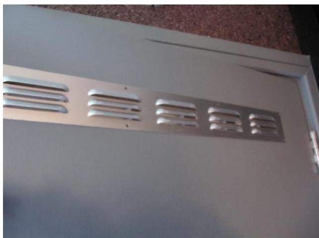
Fire door to plant room is fitted with high and low level air vents, in the event of fire starting in the plant room these would allow fire and smoke to affect the escape route from the public areas.
